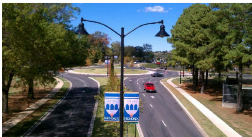
Figure 4-2 Two Lane Roundabout Example
