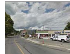
B2-33 Proposed Sign Location 1. Install Downtown Directional T-2 with right arrow and Parking Lot Directional T-1 with right arrow. 2. Install both signs on same post if possible.
