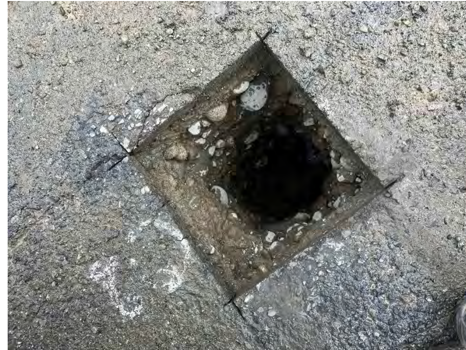
Photograph 2: View of TH23-02; typical view of hydrovac test hole from surface.
