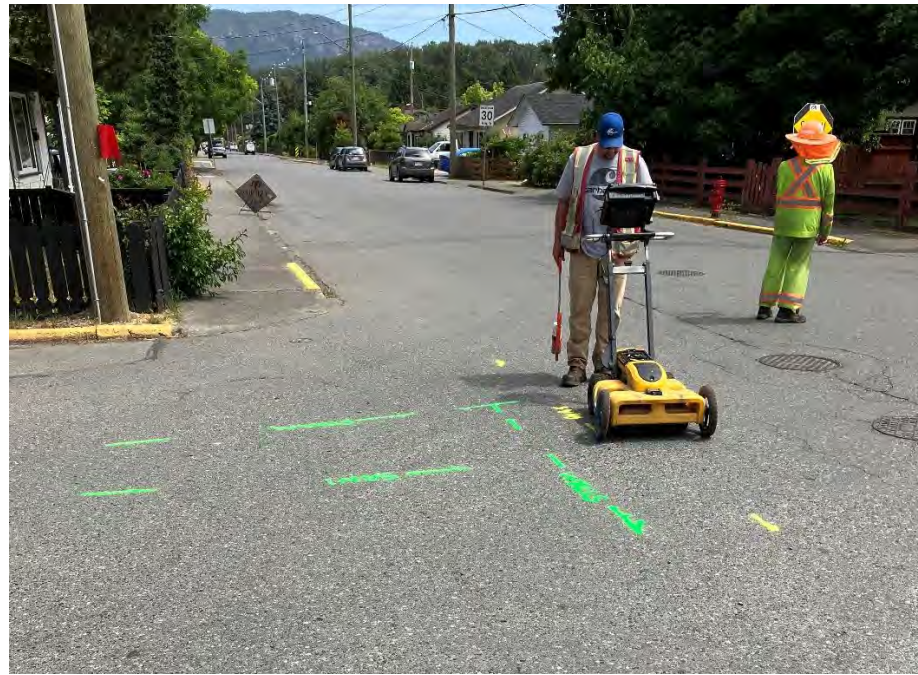
Photograph 1: Utility locating activities on Marchmont Rd at Day Rd.
