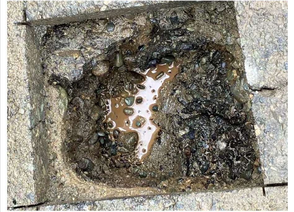
Photograph 3: View of asphalt fill material encountered at TH23-03.
