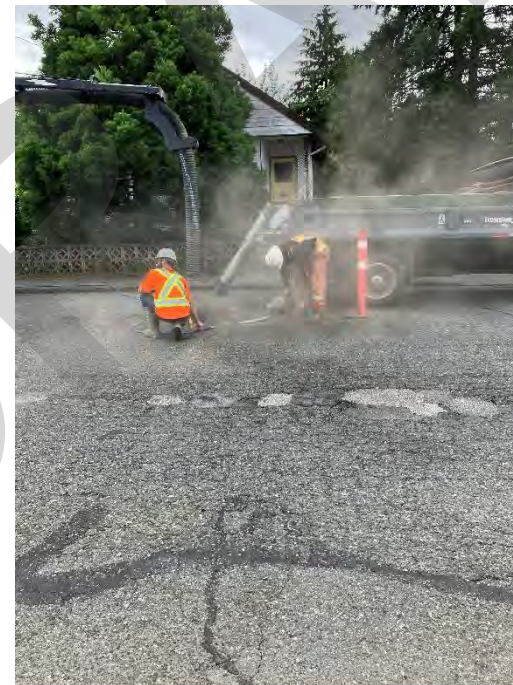
Photograph 5: View of Hydroforce sawing through the asphalt at location TH23-03.
