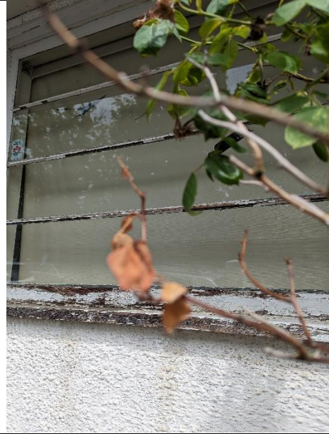
Sample: 50288 – 32 Location: Exterior – Window – South Description: Window Putty Asbestos: None detected
