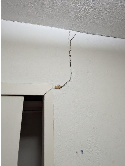
Sample: 50288 – 3 Location: Bedroom 1 – Wall Description: Drywall Joint Compound/Textured Coating Asbestos: Chrysotile 1%
