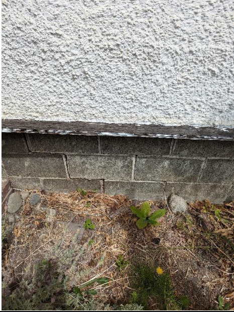
Sample: 50288 – 37 Location: Exterior – Foundation Description: Brick Mortar Asbestos: None detected
