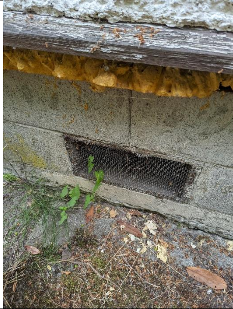
Sample: 50288 – 35 Location: Exterior – Foundation Description: Brick Mortar Asbestos: None detected
