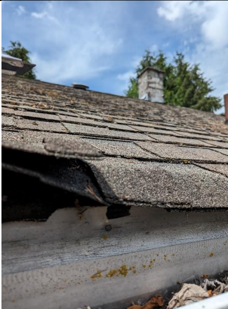
Sample: 50288 – 40 Location: Rooftop Description: Tar Shingle/Roof Felt Asbestos: None detected
