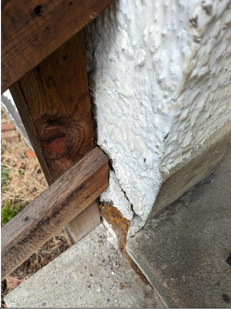
Sample: 50288 – 29 Location: Exterior – South Description: Stucco Asbestos: None detected
