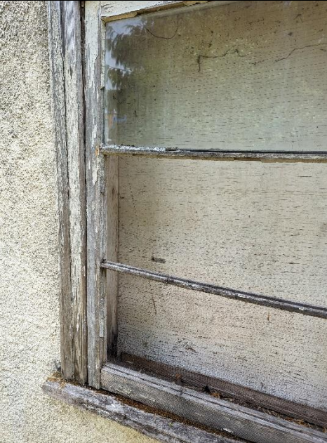
Sample: 50288 – 39 Location: Garage – Window Description: Window Putty Asbestos: None detected
