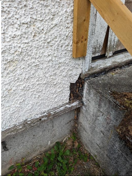
Sample: 50288 – 31 Location: Exterior – North Description: Stucco Asbestos: None detected
