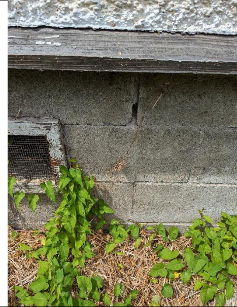
Sample: 50288 – 36 Location: Exterior – Foundation Description: Brick Mortar Asbestos: None detected
