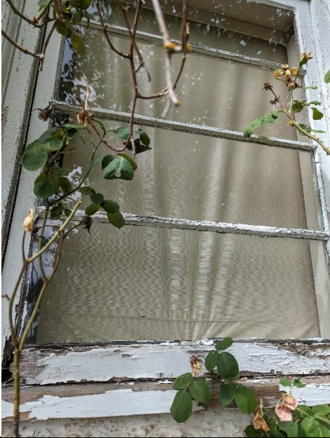
Sample: 50288 – 33 Location: Exterior – Window – Southeast Description: Window Putty Asbestos: None detected
