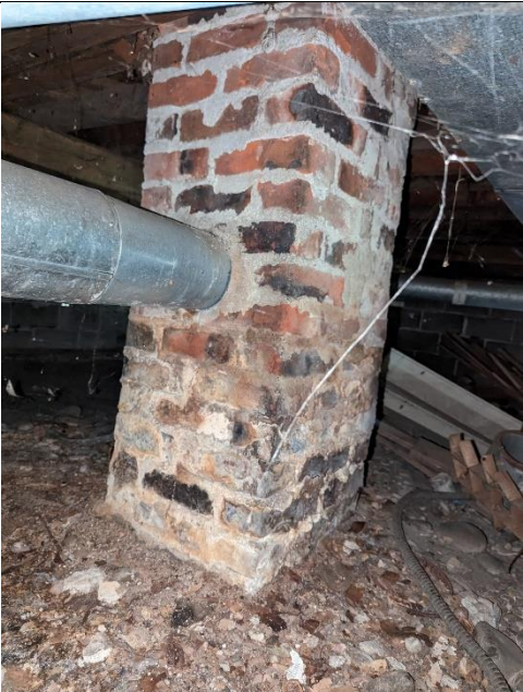
Sample: 50288 – 43 Location: Crawlspace – Chimney Description: Brick Mortar Asbestos: None detected
