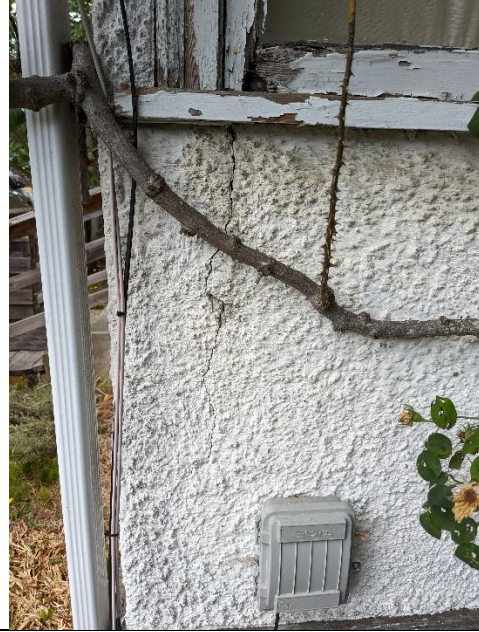
Sample: 50288 – 30 Location: Exterior – Southeast Description: Stucco Asbestos: None detected
