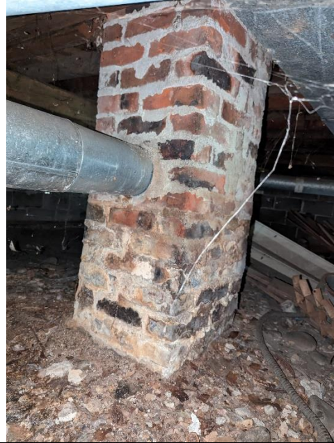
Sample: 50288 – 42 Location: Crawlspace – Chimney Description: Brick Mortar Asbestos: None detected
