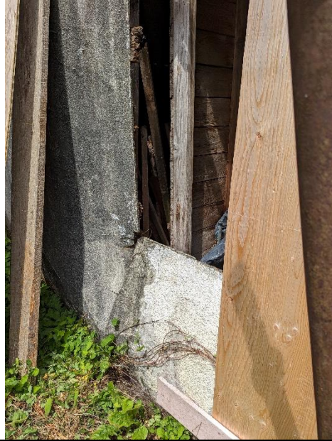
Sample: 50288 – 38 Location: Garage – Exterior Description: Stucco Asbestos: None detected
