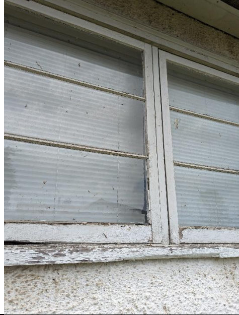
Sample: 50288 – 34 Location: Exterior – Window – East Description: Window Putty Asbestos: Chrysotile 6%
