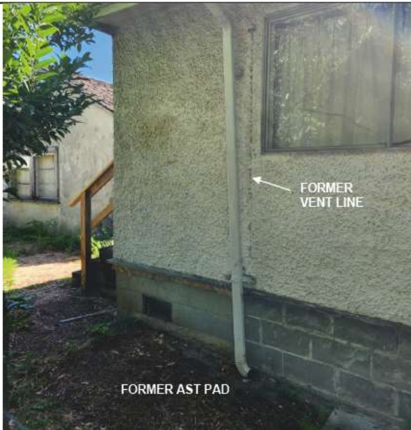
Photograph 6 Photo showing former AST pad and vent line locations at northwest corner of house.
