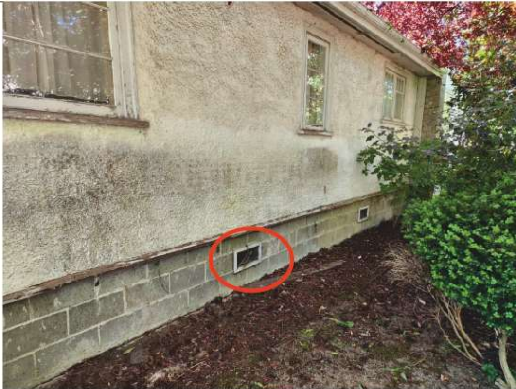
Photograph 7 Photo showing the heating oil AST supply lines, located on the west side of the house.
