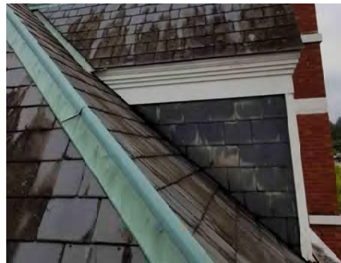
5 SLATE CLADDING TO SLOPED ROOF - PHOTO
