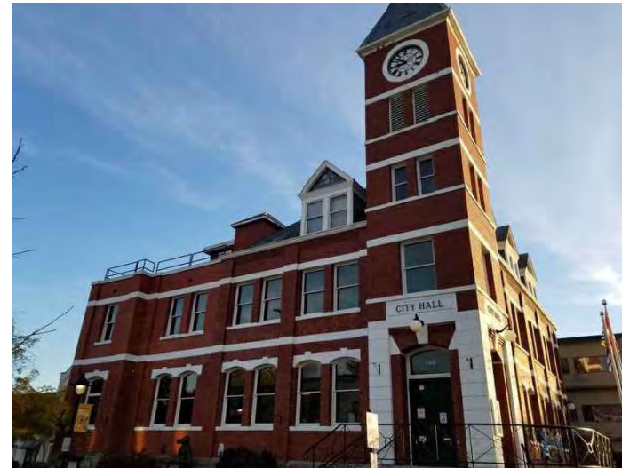
2 EXISTING SOUTH ELEVATION - PHOTO BE.000
