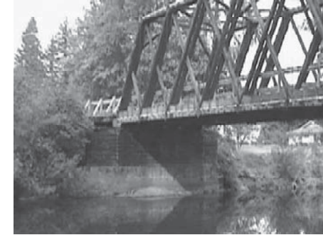
The Crofton Road Bridge over the Chemainus River.
