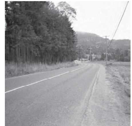
Cyclist must share this roadway as there is no paved shoulder.
