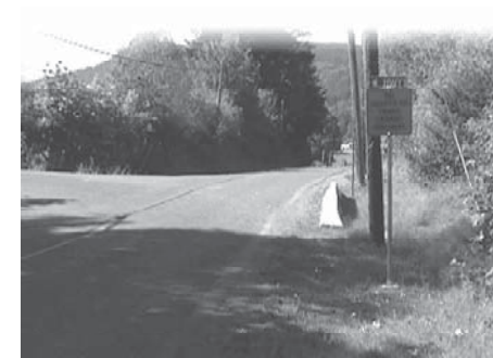
This country road is a commuter route frequently used by cyclists. This road should be upgraded to include a shoulder bikeway.
