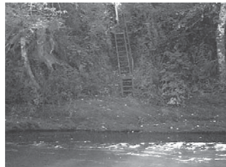
Existing stairs at Bills Road.
