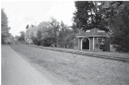
The CPR by-pass weaves around the Cowichan Station.
