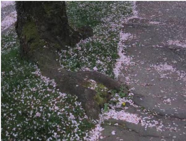
**Photo:** An example of a cherry tree roots in the City of Vancouver causing sidewalk damage
