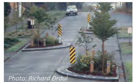
EXAMPLE: Chicanes on a narrow shared street provide traffic calming and space for planting.
