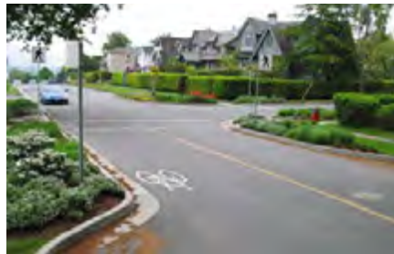
EXAMPLE: On low-volume residential streets, many communities are reducing pavement width to allow space for street trees and stormwater management components.
