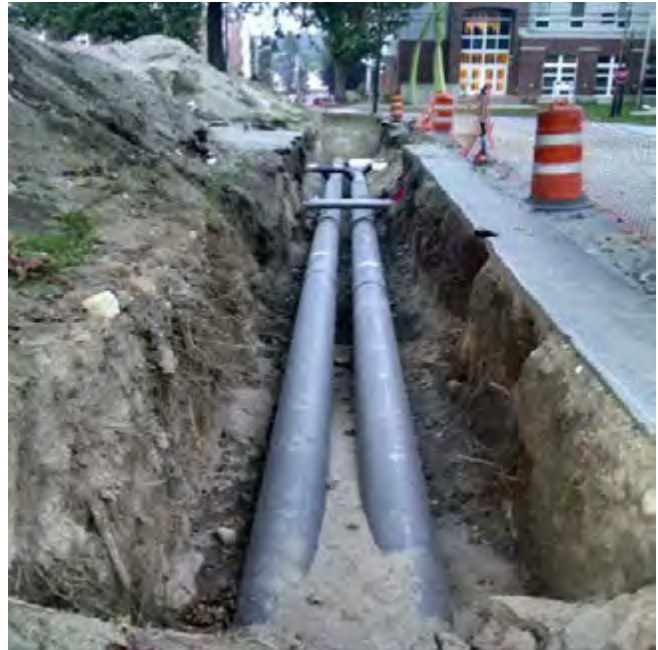
Underground utilities under construction.
