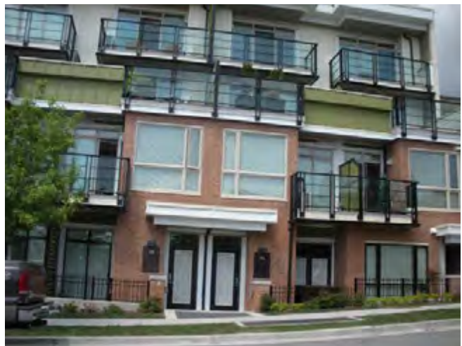
EXAMPLE. Buildings that step back on the third and fourth storeys help reduce the mass of the building and limit shading impacts. Setbacks also provide outdoor living spaces for upper residential units.
