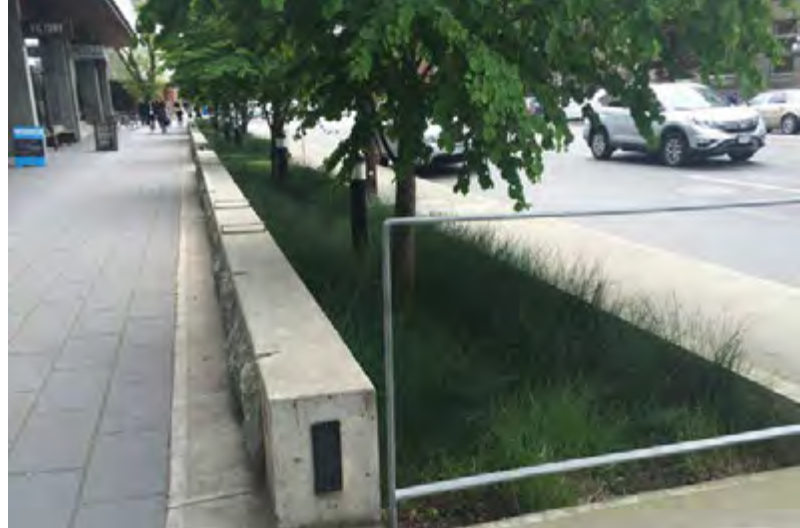
A stormwater swale in a downtown street
